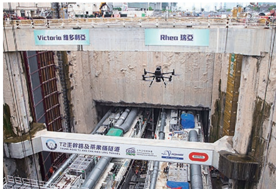
■ 運用邊緣人工智能及傳感器融合的智能隧道表面檢測系統 Edge-AI powered multi-sensor aerial inspector for tunnel surface
